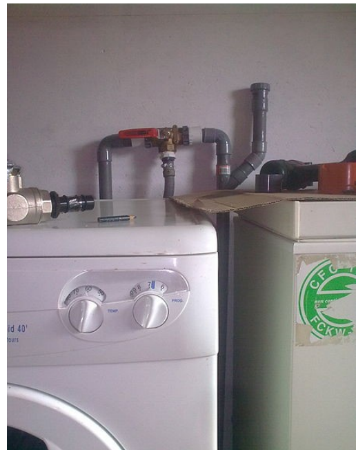
Three-way valve on a laundry-to-landscape system Image: Sustainable Sanitation Alliance
