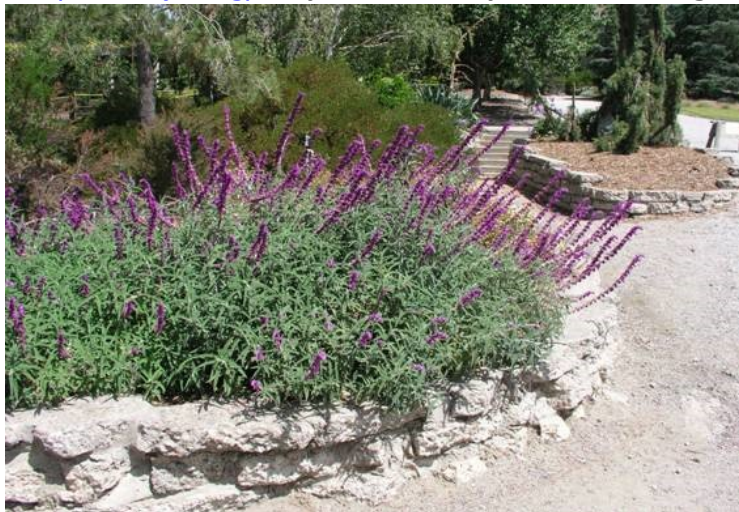
Example of a low-waste landscaping. Reused concrete retaining wall serves as a planter for a "hedge" that does not require pruning. Beds and walkways that could have been turf are gravel and mulch.
